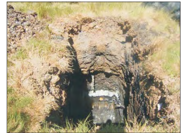
TP 21 viewed from the south
